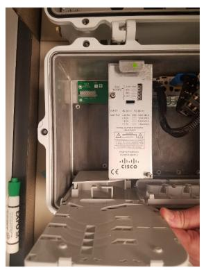
**3.** Plug in a spare power supply into the redundant slot, tighten the two retention screws and let the node sit for 2 minutes to achieve power stability.
